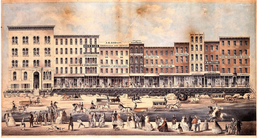
Raising a block of Chicago buildings (Edward Mendel, 1857)
